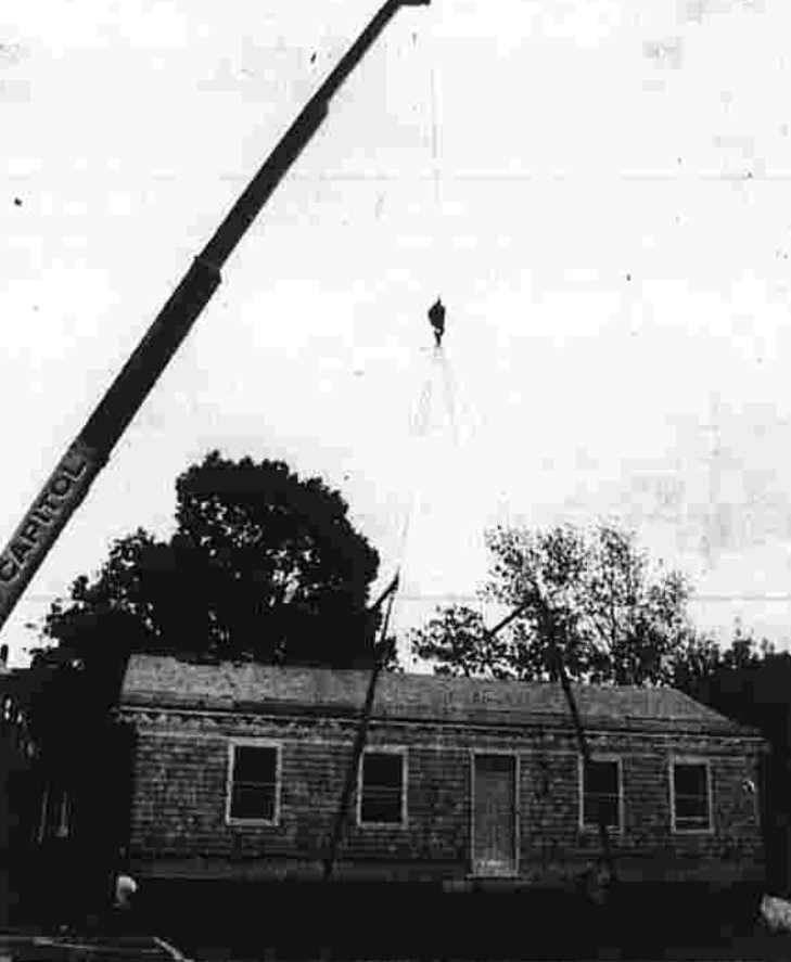
New energy saving modular home being erected at ERA Lescapance Agency at 457 Center St., Manchester.
